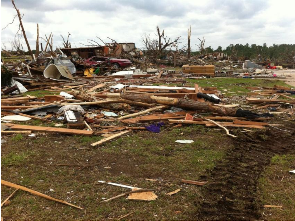
Figure 8.2 Wall and roof partially damaged at the outer edge of the Joplin tornado path
