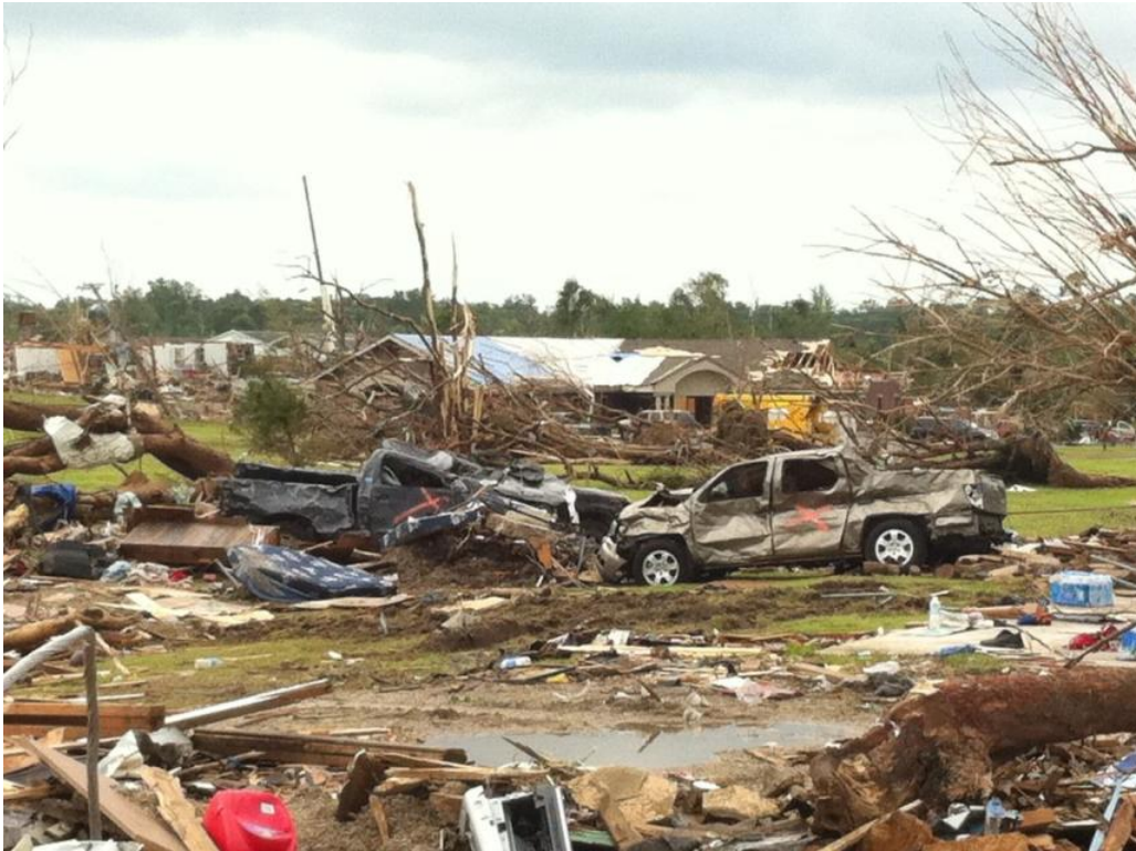
Figure 8.1 Roof and wall partially damage at the outer edge of the Joplin tornado path
